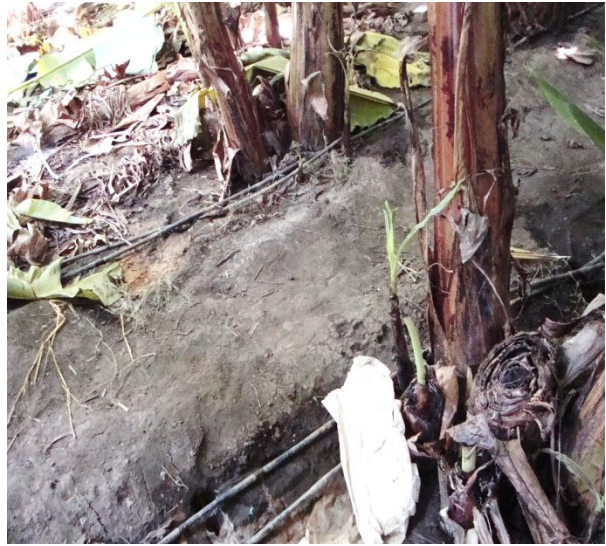
Drip irrigation in the same plantation (now producing)
