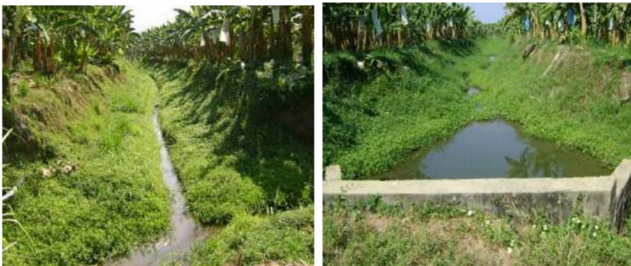
Figure 22 - 23. Main drainage channels
