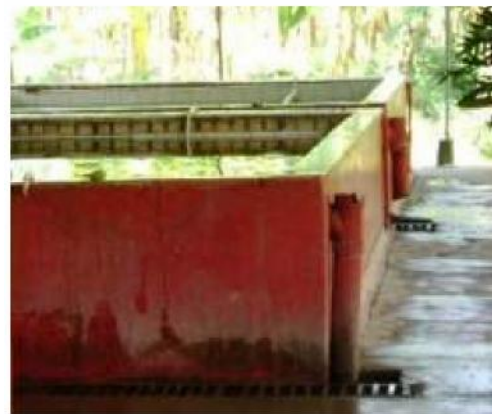
Figure 53. Packing plant floors
