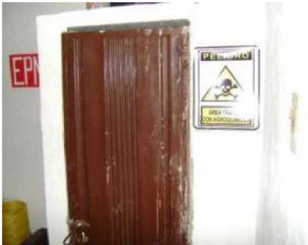
Figure 9. Agrochemical storage room
