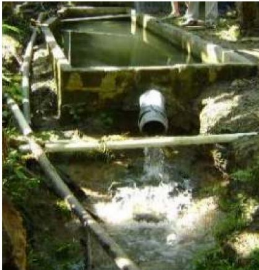
Figure 2. Collecting water for fruit washing and irrigation by gravity.
