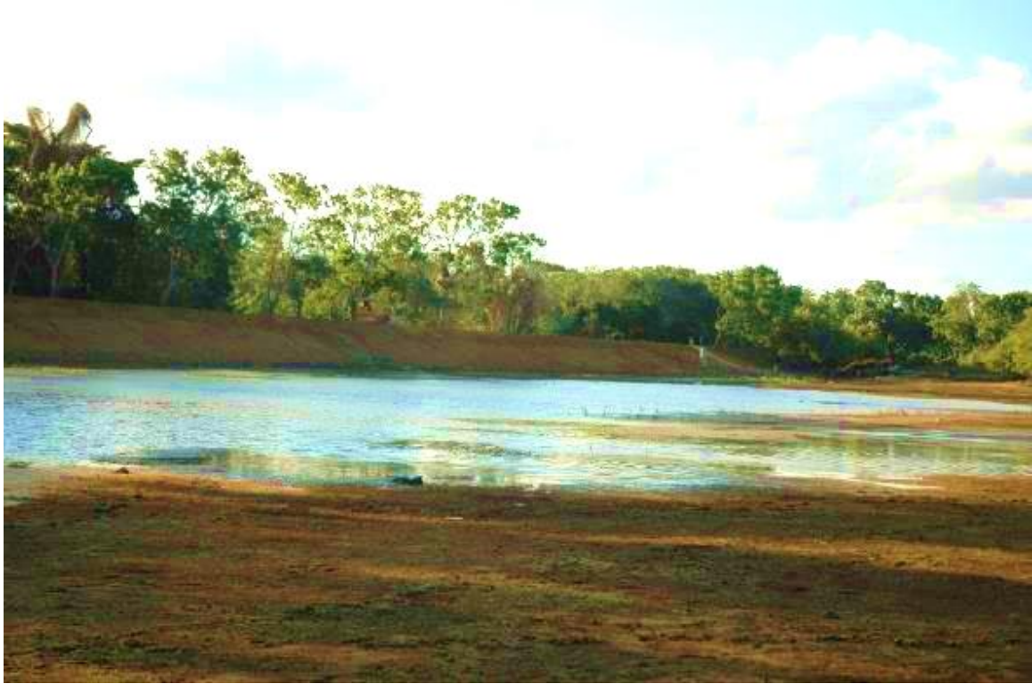
Figure 53: A Tank bund
