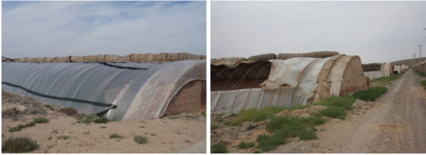
Fig. 18.4 The greenhouses provided by EPs in Bayanhuode resettlement village. The picture on the left was taken in the summer of 2008 when resettled herders were starting to learn vegetable cultivation, and the picture on the right was taken in summer of 2010, showing most greenhouses had been abandoned.
