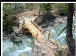
67 wooden bridge constructed
