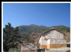
28 Community buildings constructed
