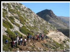
9.7 Km road constructed
