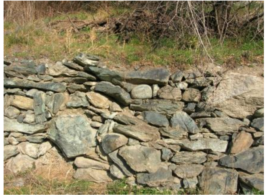
Dry Stone wall in Valle d'Aosta – NW Italian Alps
