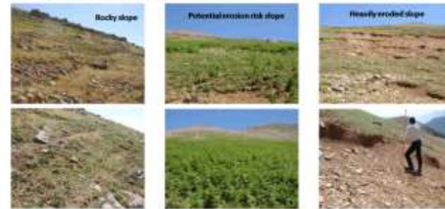
Slope area (Area2) Type of slope by erosion feature
