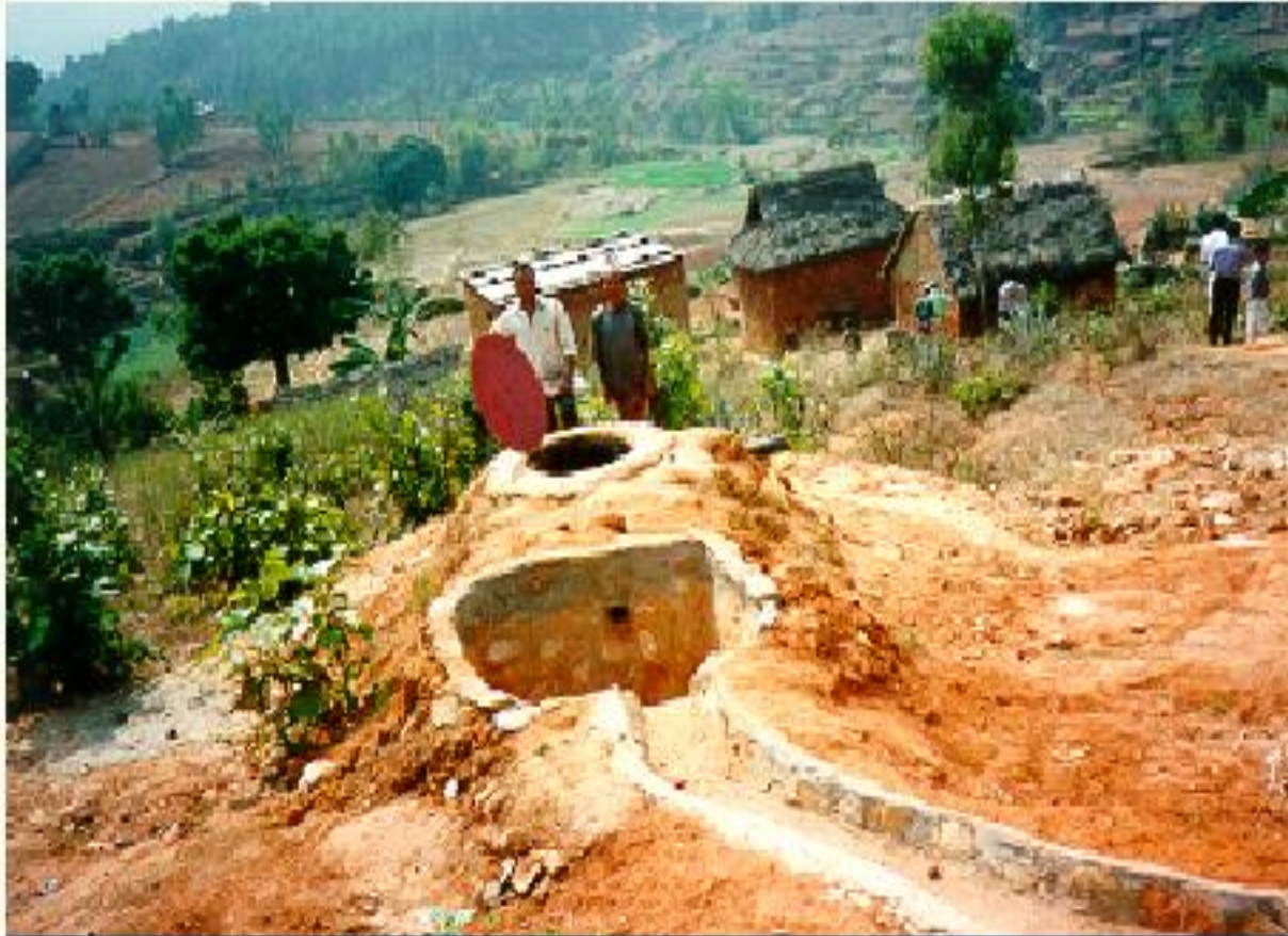
Surface water runoff collection system with sediment trap. Monsoon rain is stored for drip irrigation during dry season (Nepal)
