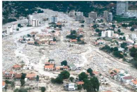
Figure 14. Debris-flow damage to the city of Caraballeda, located at the base of the Cordillera de la Costan, on the north coast of Venezuela. In December 1999, this area was hit by Venezuela's worst natural disaster of the 20th century, several days of torrential rain triggered flows of mud, boulders, water, and trees that killed as many as 30,000 people. (Photograph by L.M. Smith, Waterways Experiment Station, U.S. Army Corps of Engineers.)
