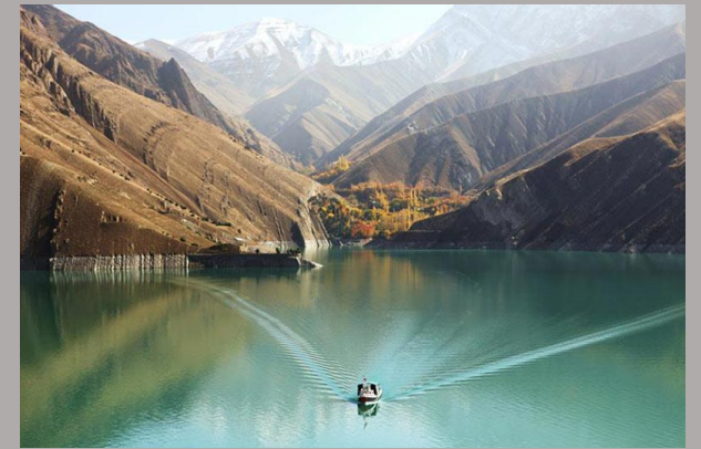
Amirkabir Dam in Central Alborz
