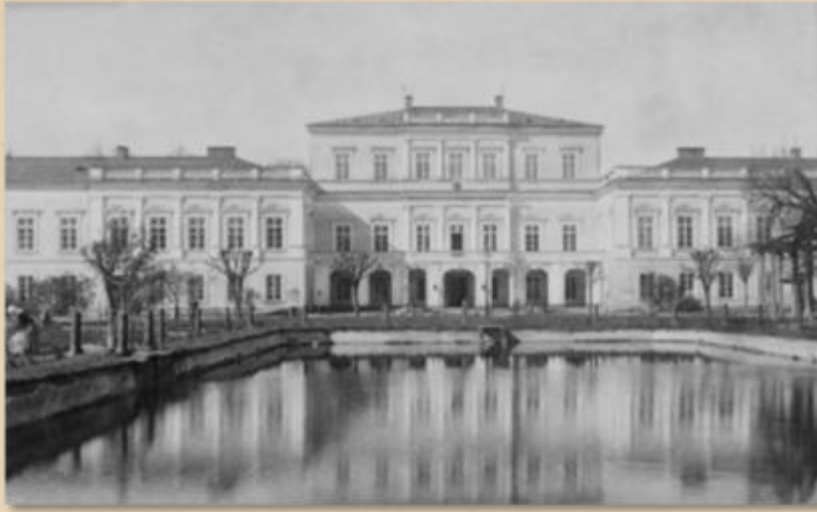
The main building of the New Alexandria Institute. Photo from the album. CSM GIK №2-9
