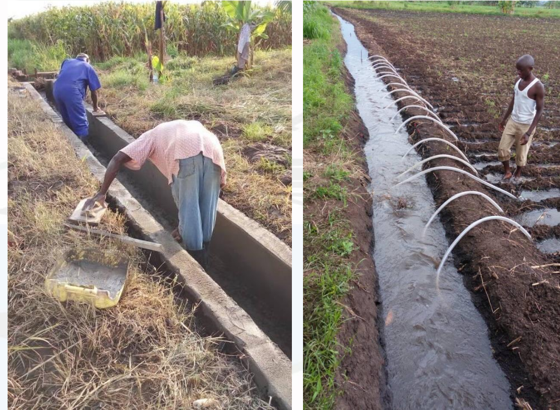
Fig.8: Improved Tertiary and Field Canals.
