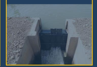
Calibrated modules a masques at tertiary level controlled manually by the farmers after irrigation rotation
