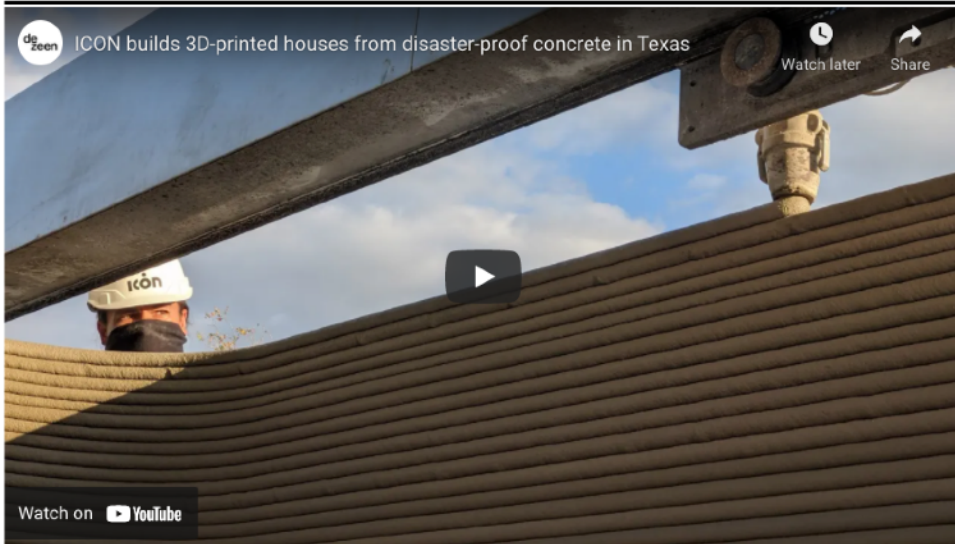
ICON builds 3D-printed houses from disaster-proof concrete in Texas
