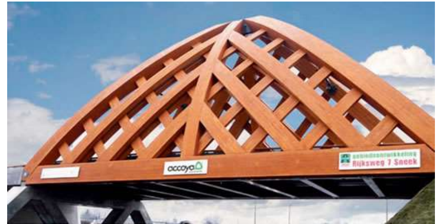
Accoya acetylated timber bridge is expected to last 50 years
