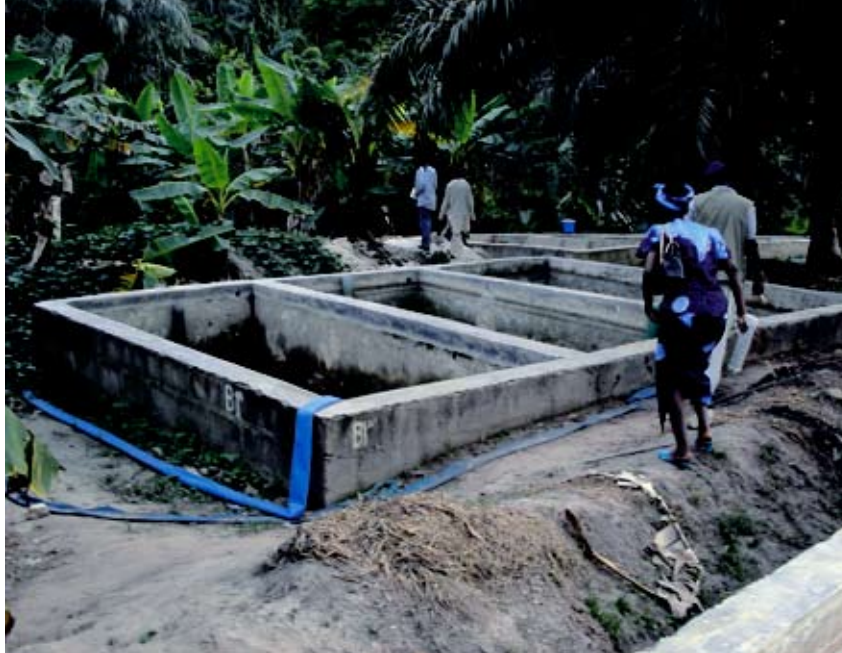
Simple static-water cement-block tanks in Nigeria produce high yields
