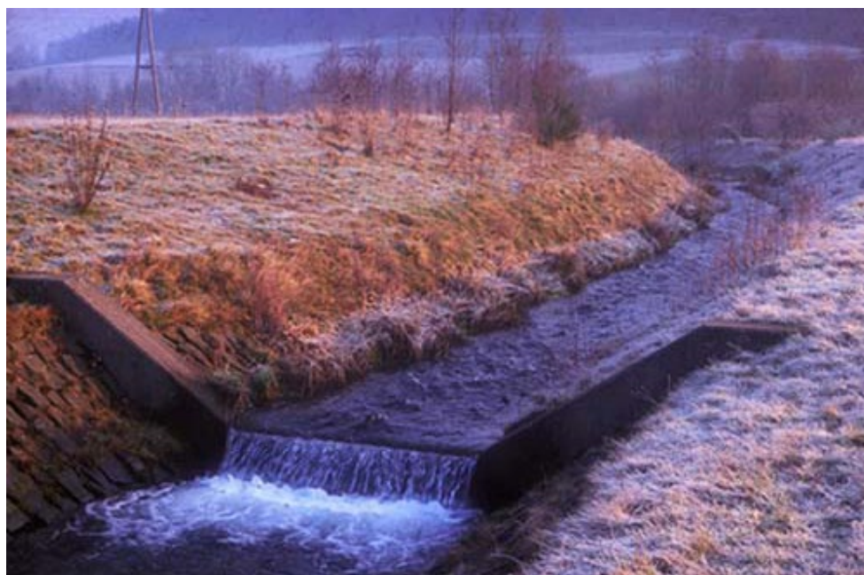
Photo 4: Even low cross-river sills can constitute obstacles depending on the swimming capacities of the fish species concerned. (Photo: G. Marmulla).
