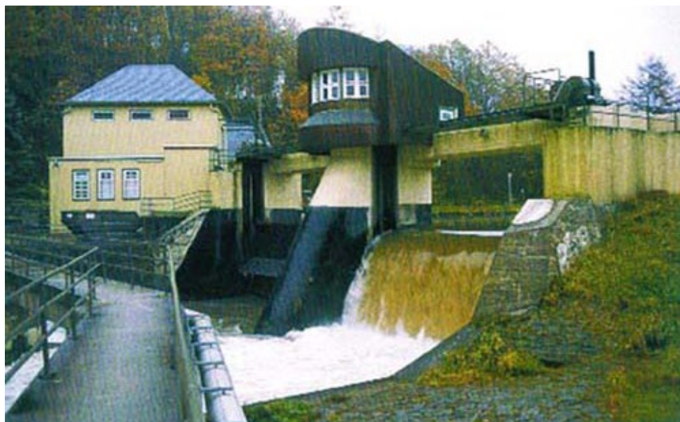
Photo 3: Dams and weirs, regardless of their height, block fish passage if not equipped with well-functioning fish passage facilities for upstream and downstream passage. The photo shows the weir of a hydropower station on a tributary to the river Rhine where Atlantic salmon once was common. (Photo: G. Marmulla).
