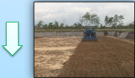
9. Levelling & Compacting
