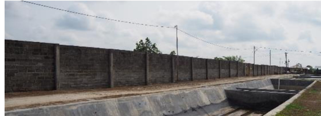
A farm with surrounding wall
