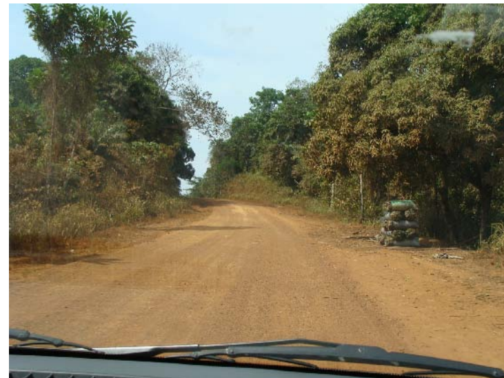
Figure 7-1 Laterite or unpaved roads
