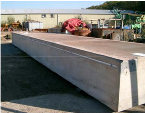
Figure 6-7 All concrete pontoon (left), Timber decked pontoon (centre) and typical pile guide for a pontoon (right)
