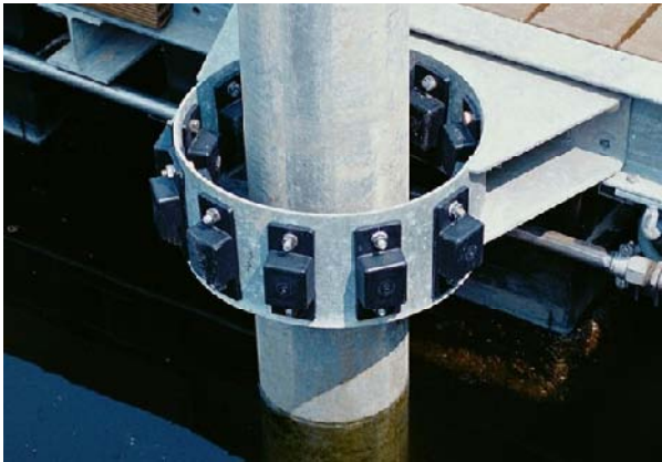
Figure 6-7 All concrete pontoon (left), Timber decked pontoon (centre) and typical pile guide for a pontoon (right)
