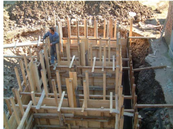
Figure 12-2 A septic tank under construction
