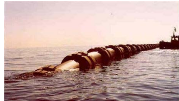
Figure 12-7 A large diameter outfall being placed – www.pipelife Norge
