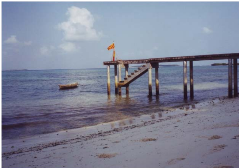
Figure 6-6 Typical piled jetties with low tide access (left)
