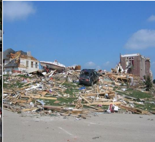
F3 Tornado Damage
