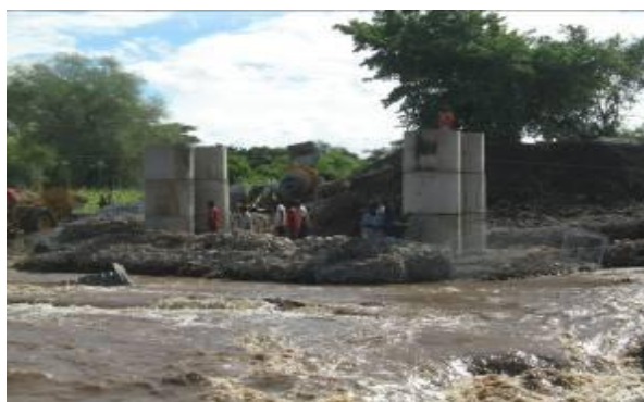
Bridge reconstruction after Flood damage.
