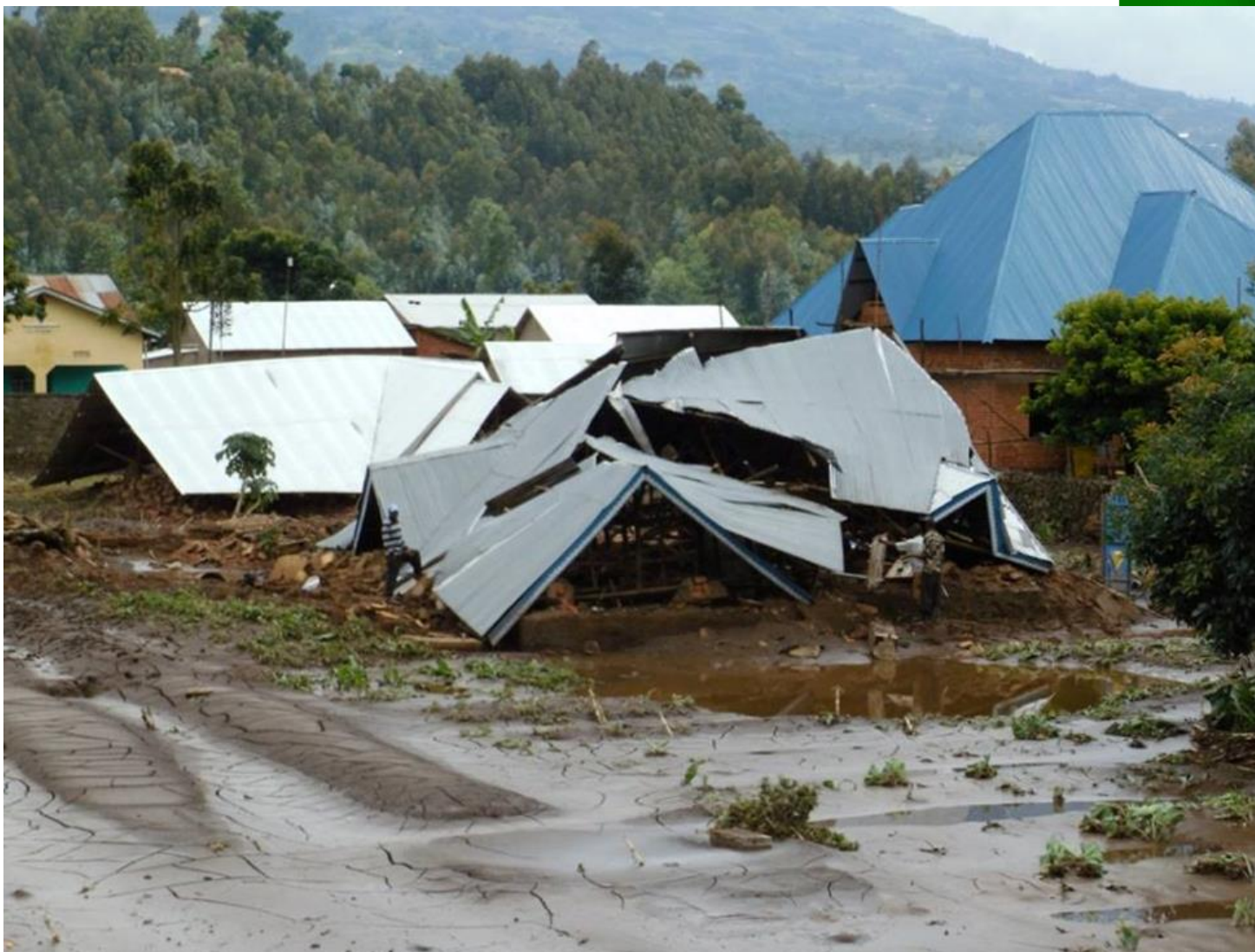
Cases of flooding damages before relocating people in high risk zones
