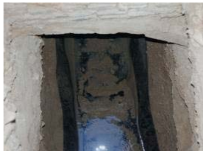
Applying geo-membrane on the gallery
