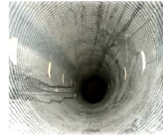
Polyethylene lining of wells
