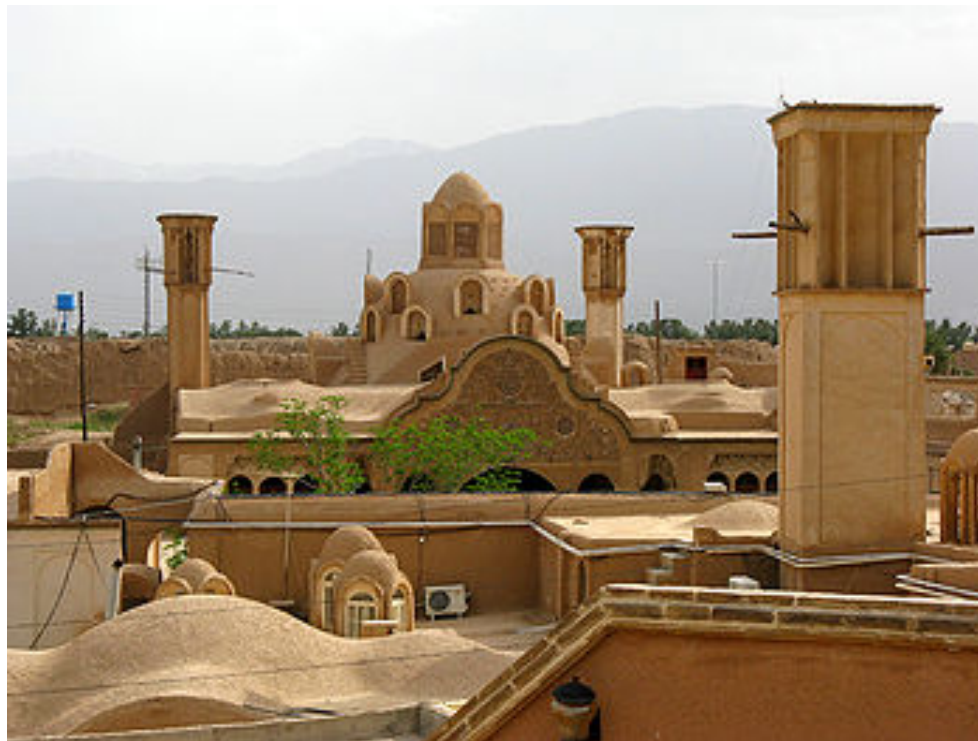
Figure 16. The wind-tower in the Brujerdis House in Kashan
